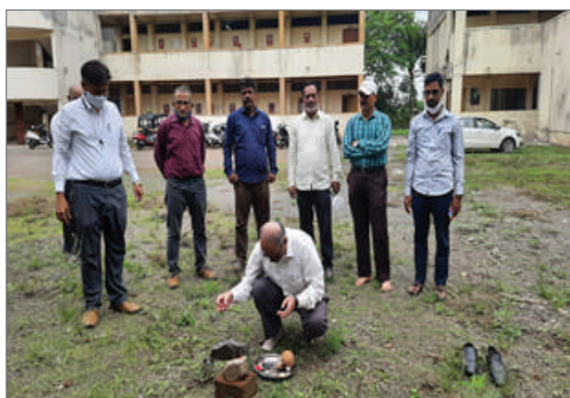
The foundation program of automatic rain gauge system
