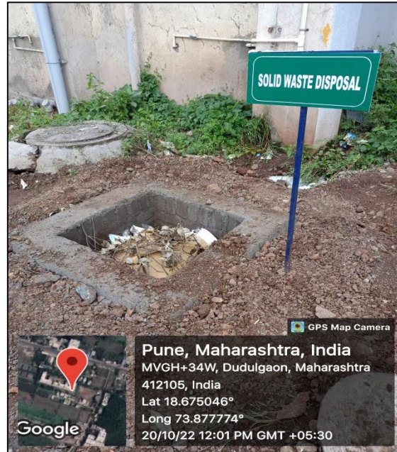
Solid waste disposal by compost pit
